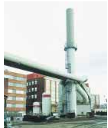
Filtering plant at melting shop
